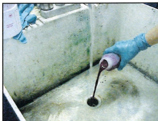
Figure 63: Dye Testing Plumbing (NEIWPCC, 2003)
